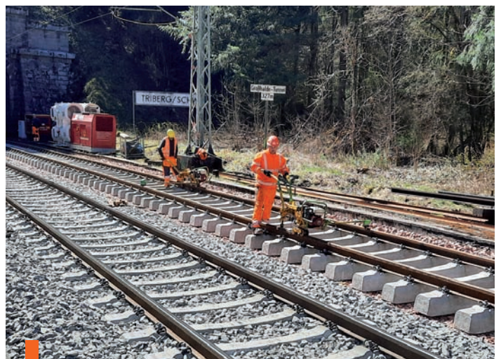
Fixing of rails (screwing)
