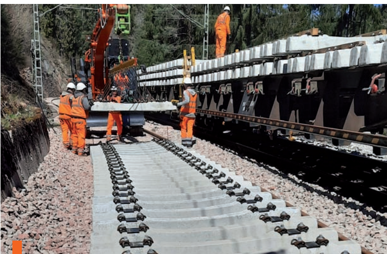
Laying of ZSX twin-sleepers by railroad excavator
