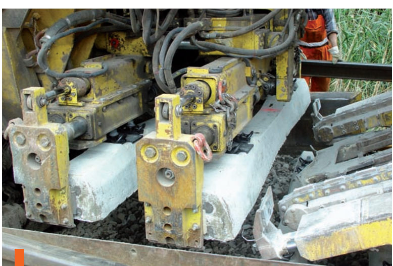
Laying ZSX with SUZ 500 UVR (double installation unit)
