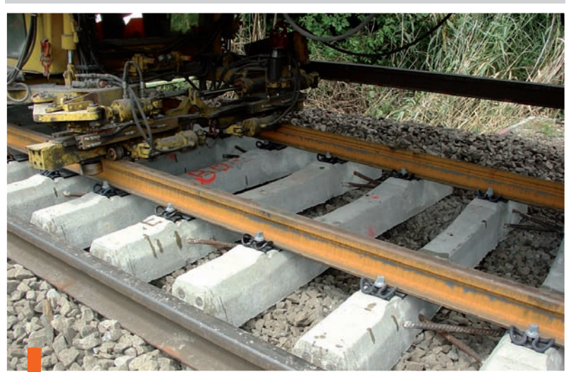
Threading of rails without moving up the sleepers
